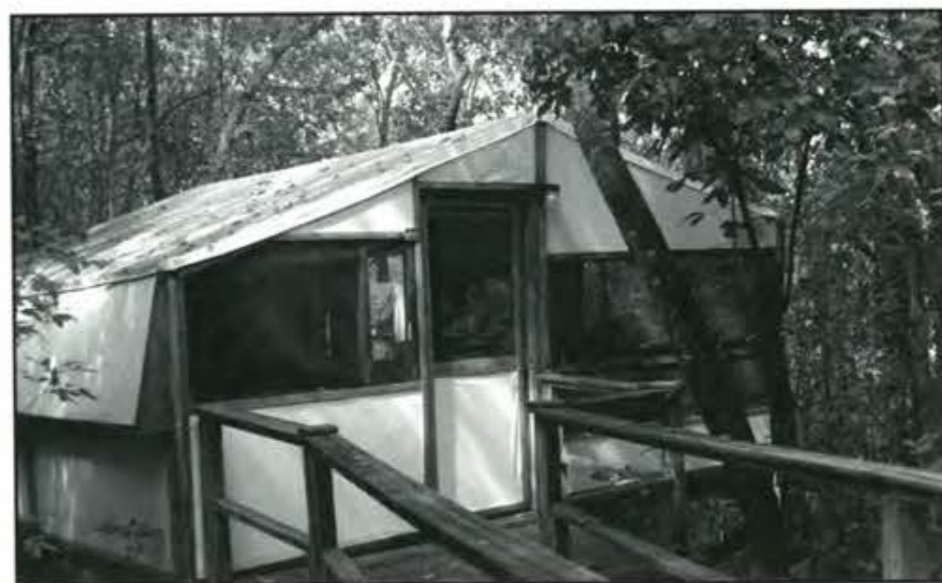
One of the 114 tent-cottages at Maho Bay Camps. The elevated walkways that connect all the tent cottages at Maho Bay prevent underlying plants and animals from being disturbed by the camp's visitors.
