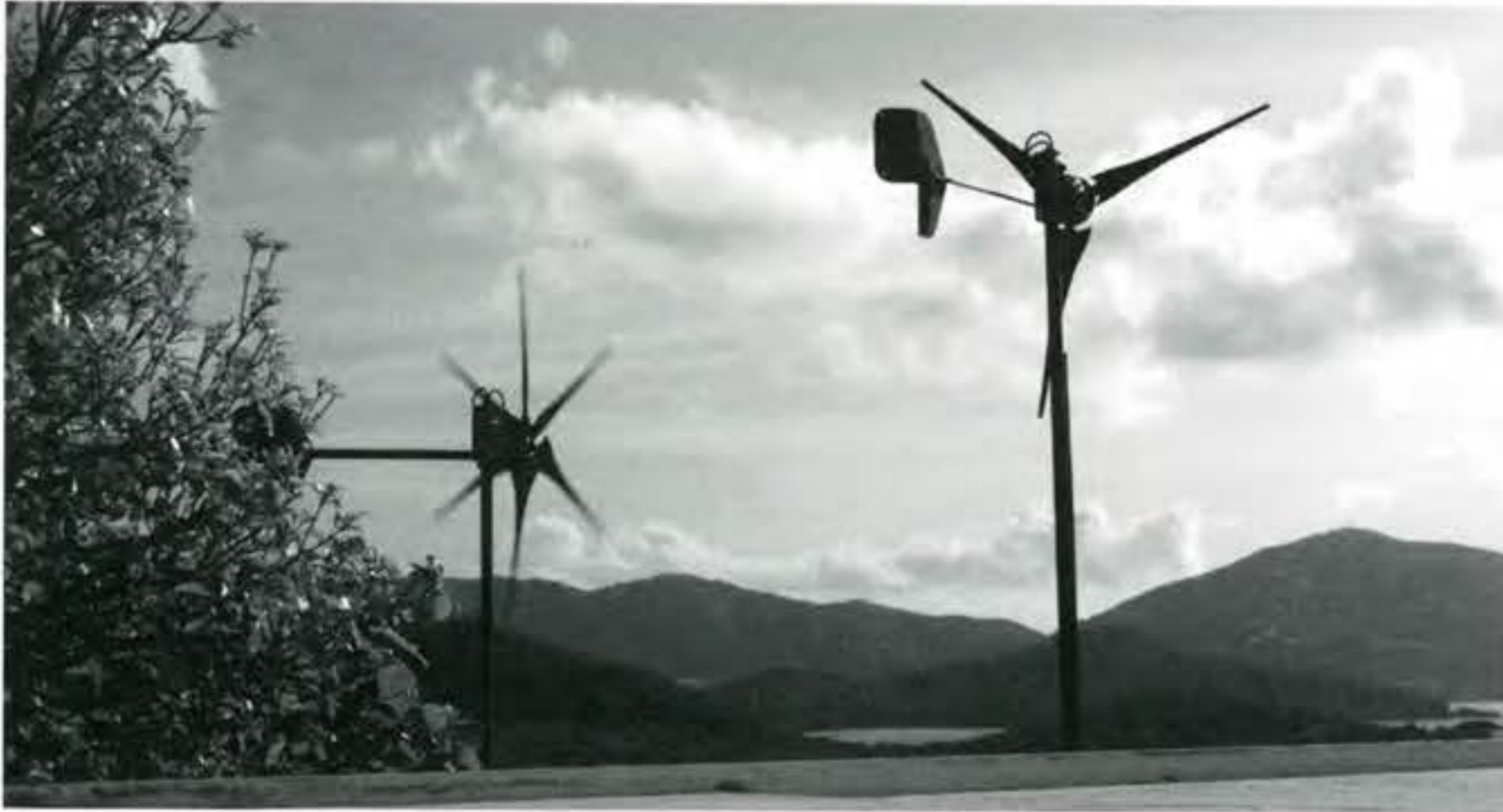
Wind turbines harness trade winds to power the communal refrigerator and lights in the four tent-cottages in the Virgin Islands Campground, Water Island, USVI.
