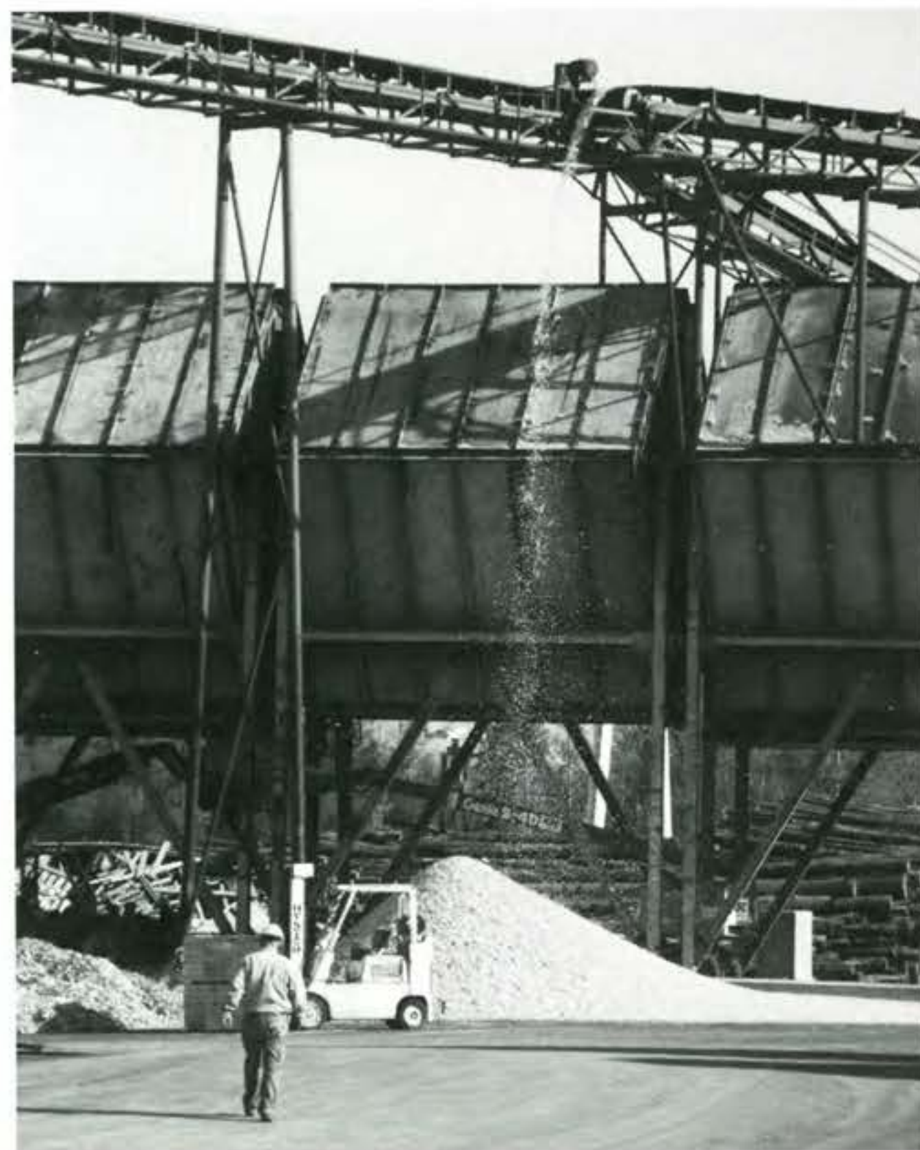
A steady stream of woodchips and sawdust cascades out of the mill, destined for the cogeneration plant. Sierra Pacific utilizes this former waste product to produce power for the site.
