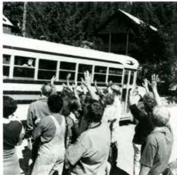
LEFT: Howe Sound Mining Co. closed the mine in 1957, but the entrance just outside the village remains open. RIGHT: Everyday a bus arrives with new villagers and departs with leaving villagers. Saying good-bye to those leaving is an important part of daily life at Holden.
