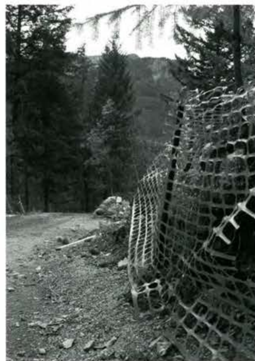
Fences protect trees from damage on the building site.
