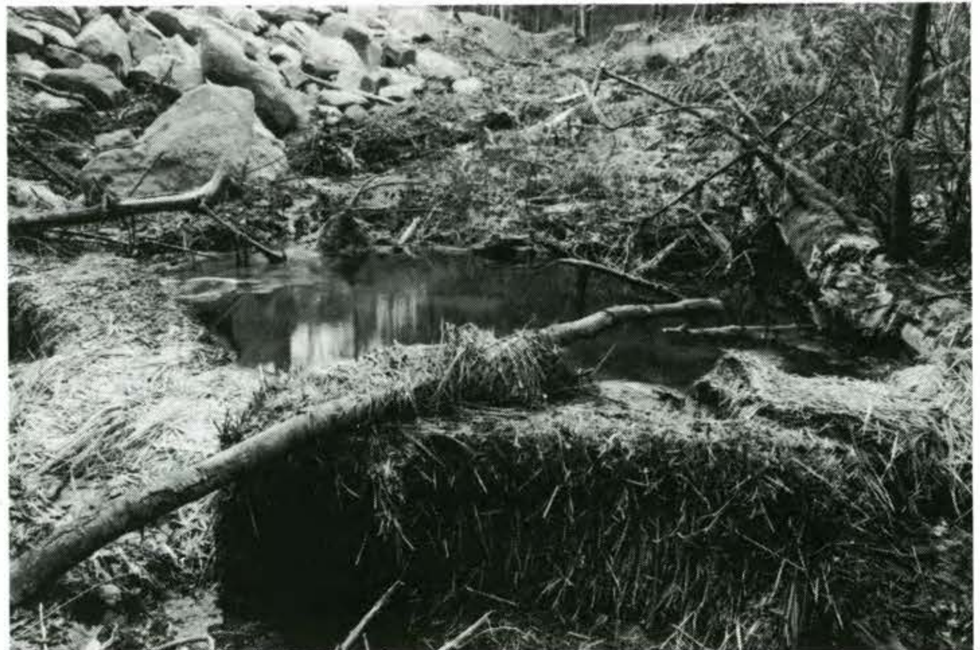
Stream rehabilitation, developer-style: hay bales in Connelly Creek.
