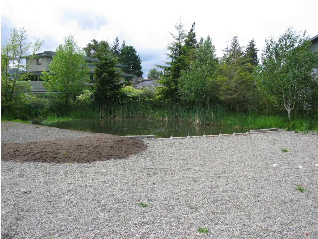
Figure A8: Photograph of the Park Place storm water treatment system in May 2006, after an extensive retrofit where two of the sites wet cells were filled with sand.
