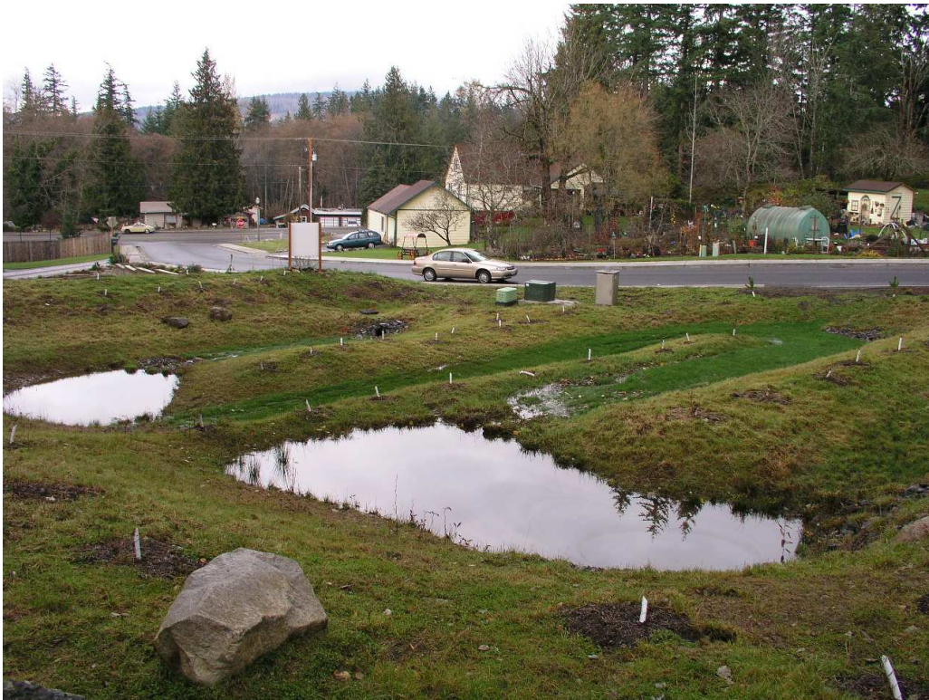
Figure A9: Photograph of the Parkstone wet pond and swale, November 2003. This site was not sampled in 2008/2009.
