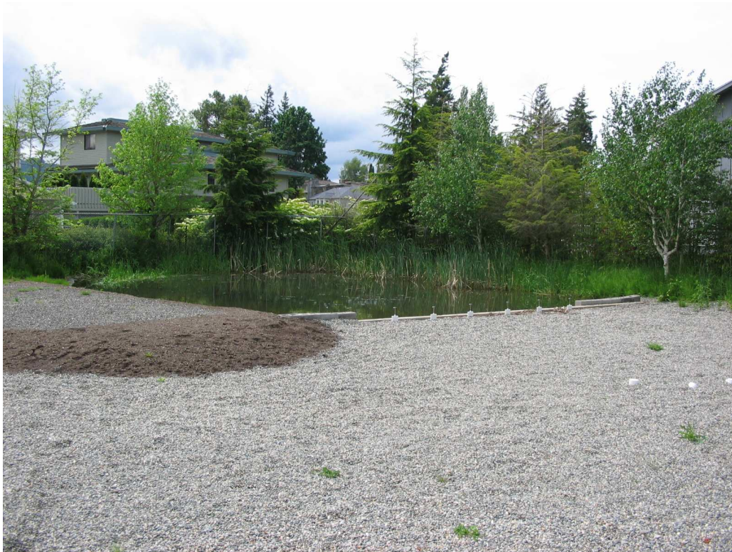
Figure A8: Photograph of the Park Place storm water treatment system in May 2006, after an extensive retrofit where two of the sites wet cells were filled with sand. This site was sampled in 2008/2009.
