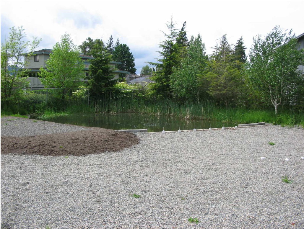
Figure A9: Photograph of the Park Place storm water treatment system in May 2006, after an extensive retrofit where two of the sites wet cells were filled with sand.
