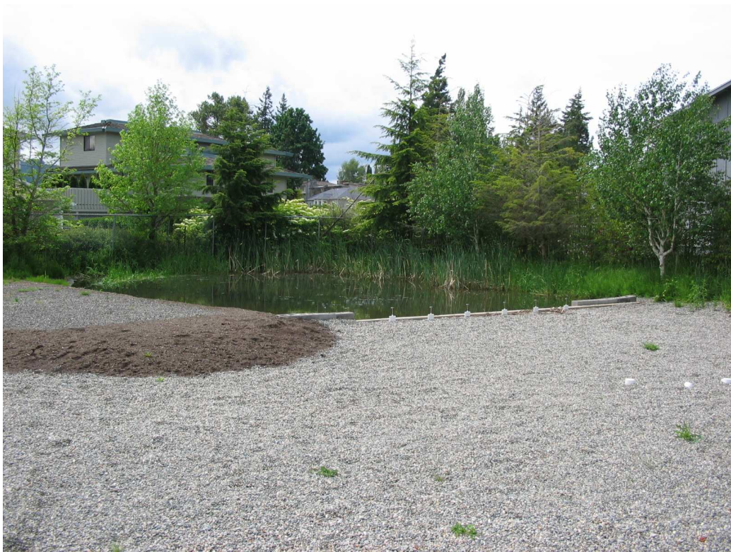
Figure A8: Photograph of the Park Place storm water treatment system in May 2006, after an extensive retrofit where two of the sites wet cells were filled with sand.
