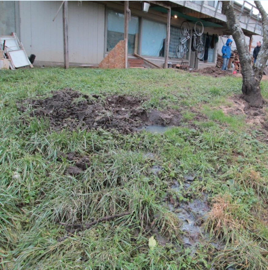
Failing drainfield
