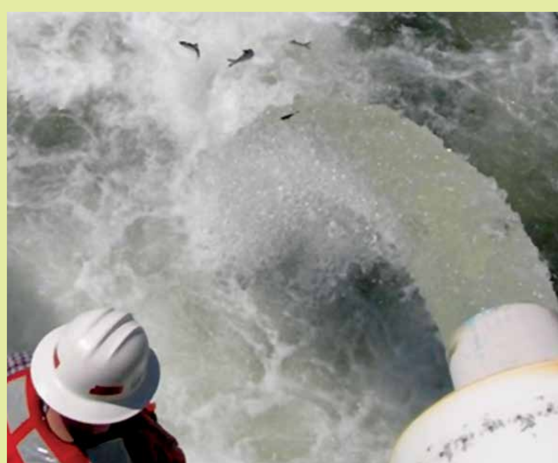
Smolt flume to get fish safely over the spillway
