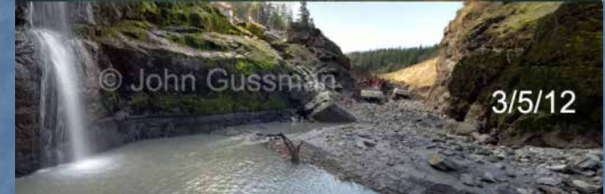
Former 105' tall Elwha Dam Removal Completed August 2012
