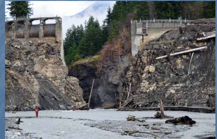
Former 210' tall Glines Canyon Dam Removal Completed August 2014
