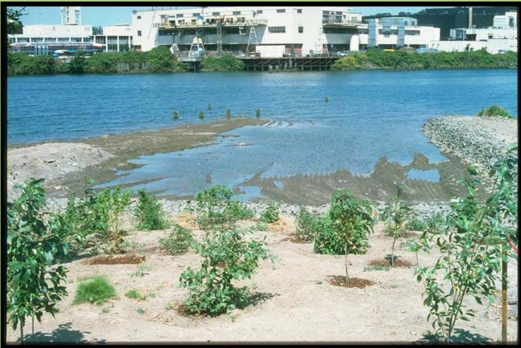
Turning Basin Number Three Demonstration Site following construction in 1996.
