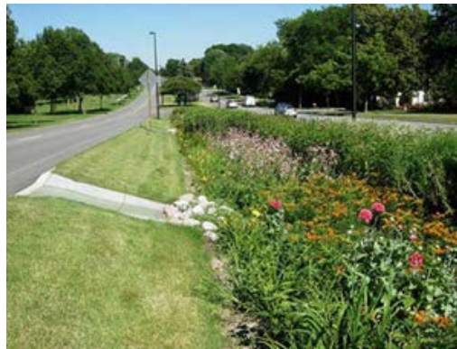
Figure 6: Example of bioswale installation. Includes depression to collect and direct rainwater to plant species that tolerate a range of moisture regimes. (Source: Science Society of America, 2018)
