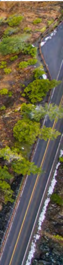
The Nooksack River flows next to Highway 542 in Washington state.
