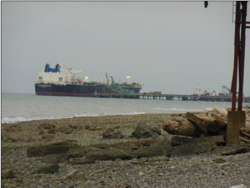
Figure 1. Photo of the current Cherry Point site including wharf and trestle (courtesy of Judith Debay).
