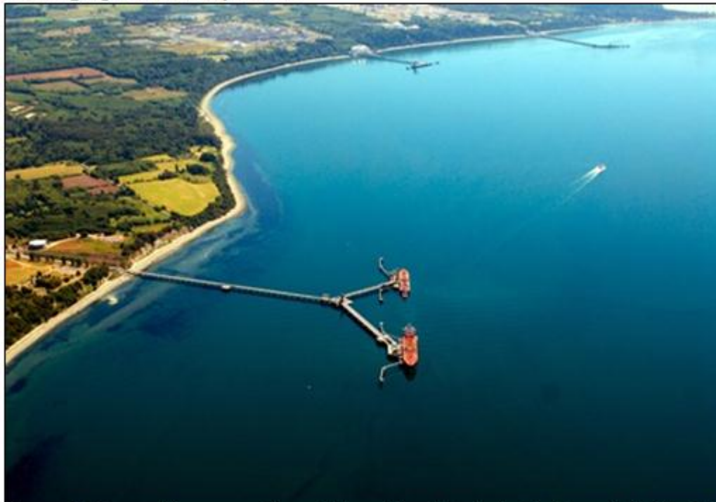
Figure 2. Photo of the current Cherry Point with original wharf and trestle (NOAA, 2009).
