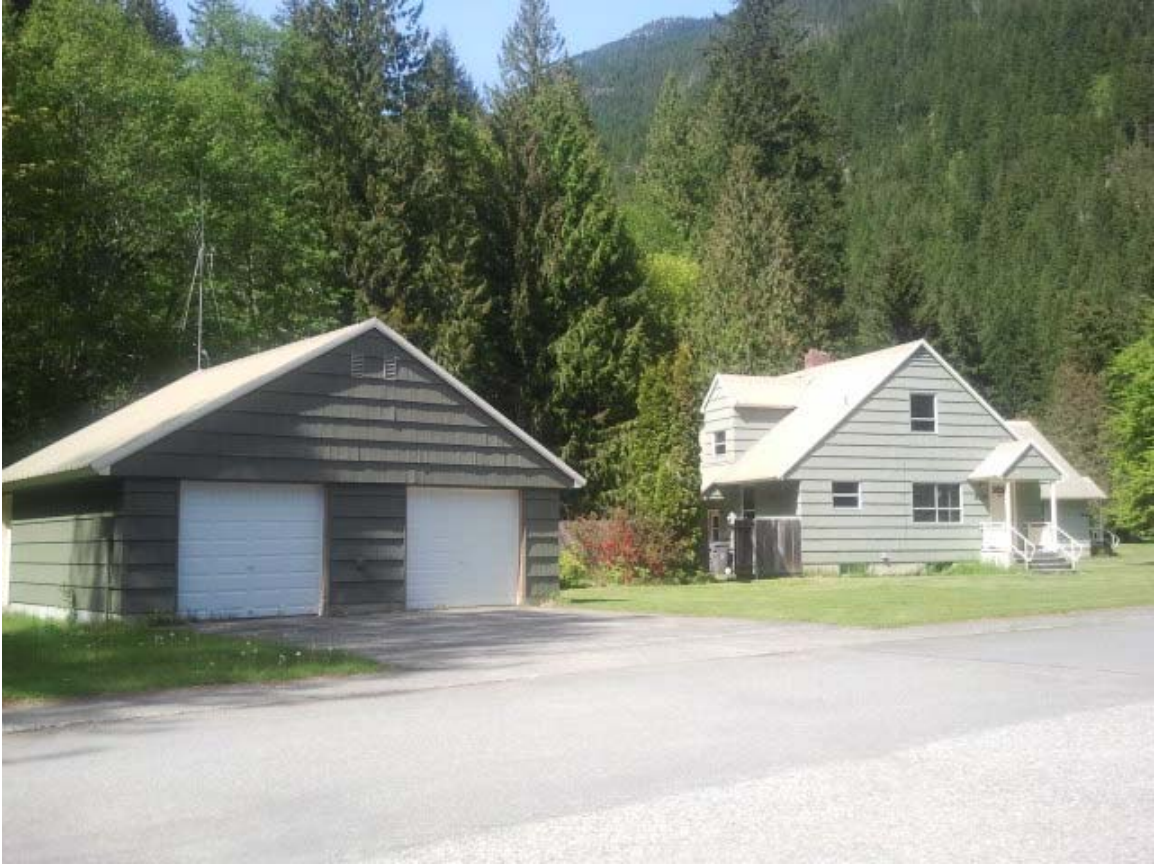
Figure 18. Displaying Garage H-1 & H-2 and Hollywood House H-1, two of the eight structures prosed for removal and relocation.
