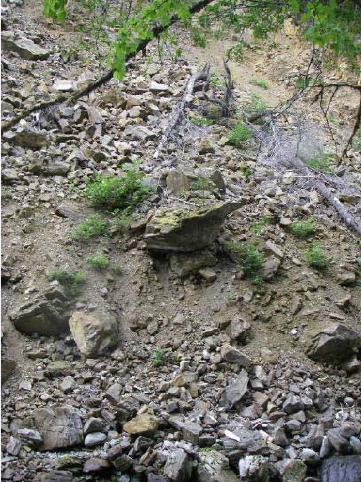
Figure 11. Image of the Stetattle Creek rockslide of 2003 (Courtesy of R2 Resource Consultants, 2013).
