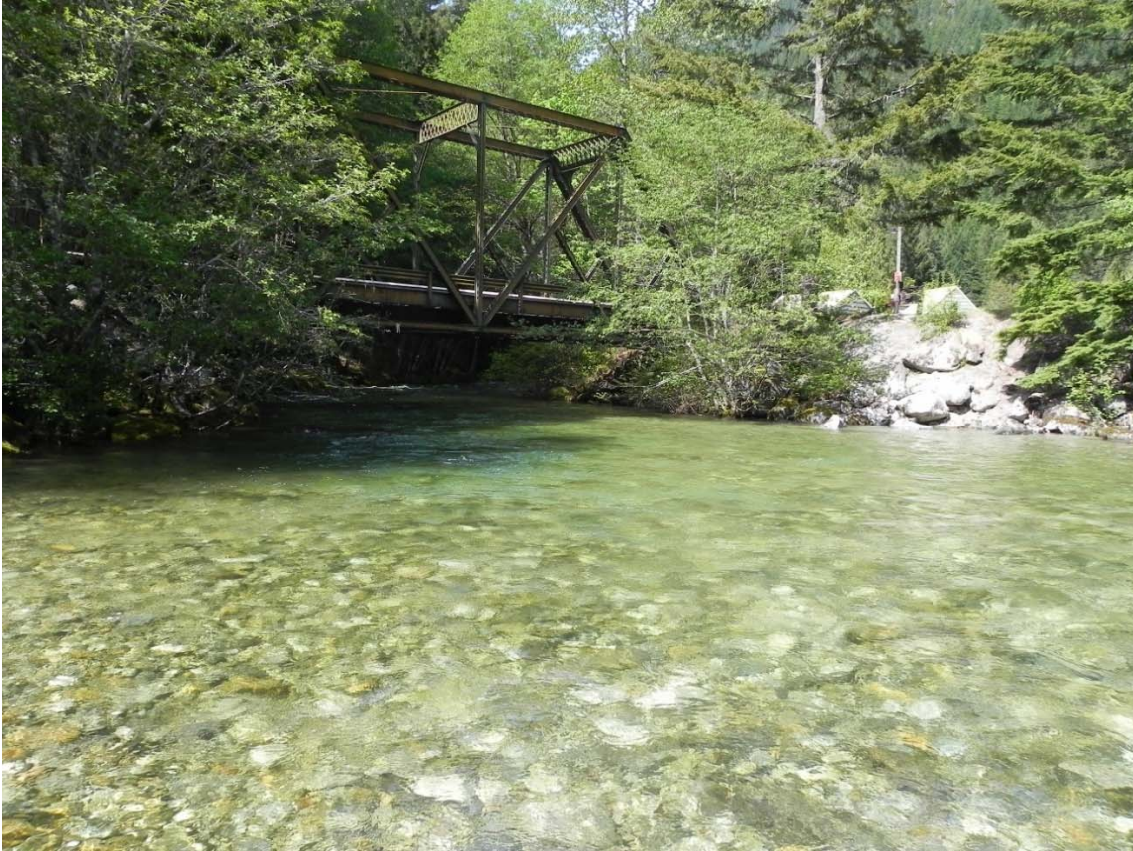
Figure 9. Image showing the mouth of Stetattle Creek, the Stetattle Creek Bridge and levee.
