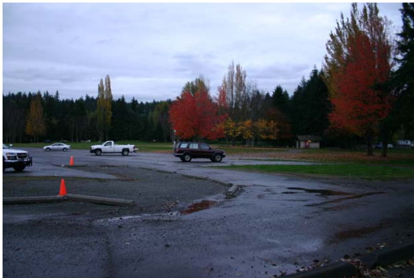
Photo 3 Existing condition of the parking lot area.
