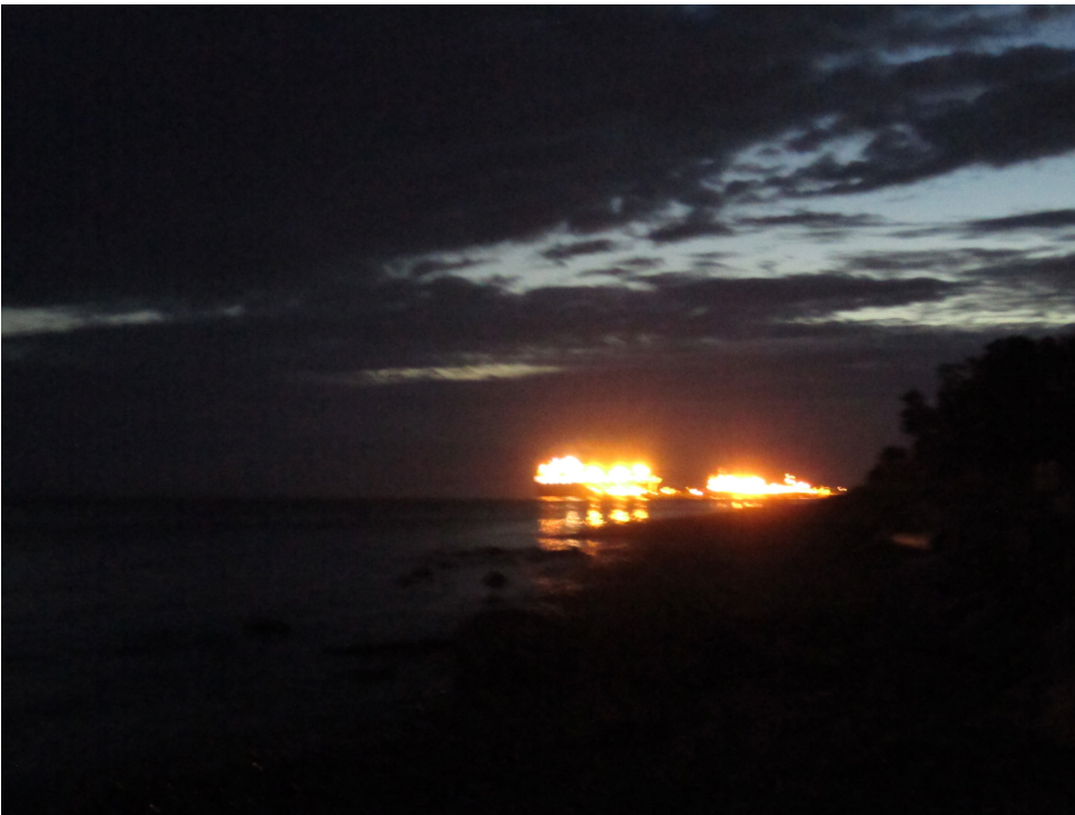
Figure 6.2 - Existing British Petroleum terminal at night
