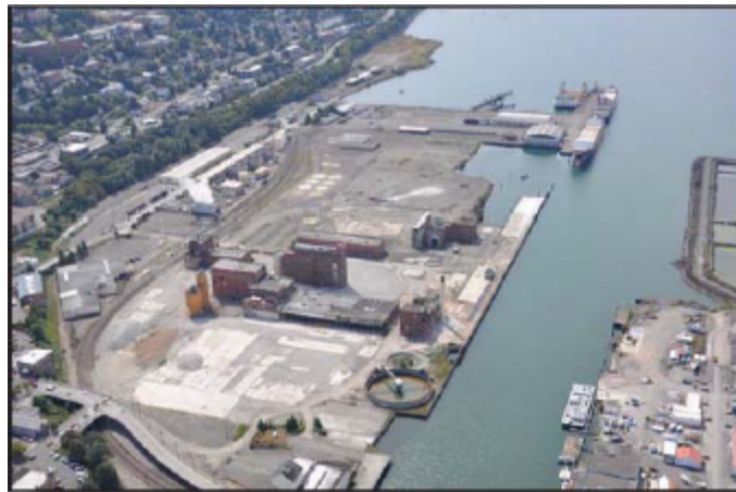
Figure 4: Remedial Action Units aerial view within the former GP West site Source: POB and COB Bellingham Public Partnership, 2013
