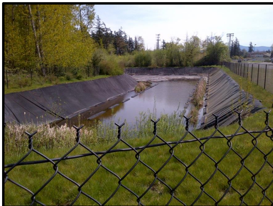
Figure 7. Photograph of Existing Stormwater Detention Pond on Alternative Site.
