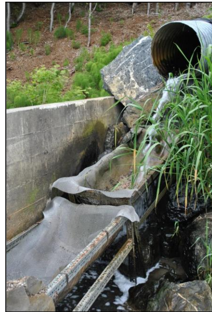
Figure 12- Outfall on Site
