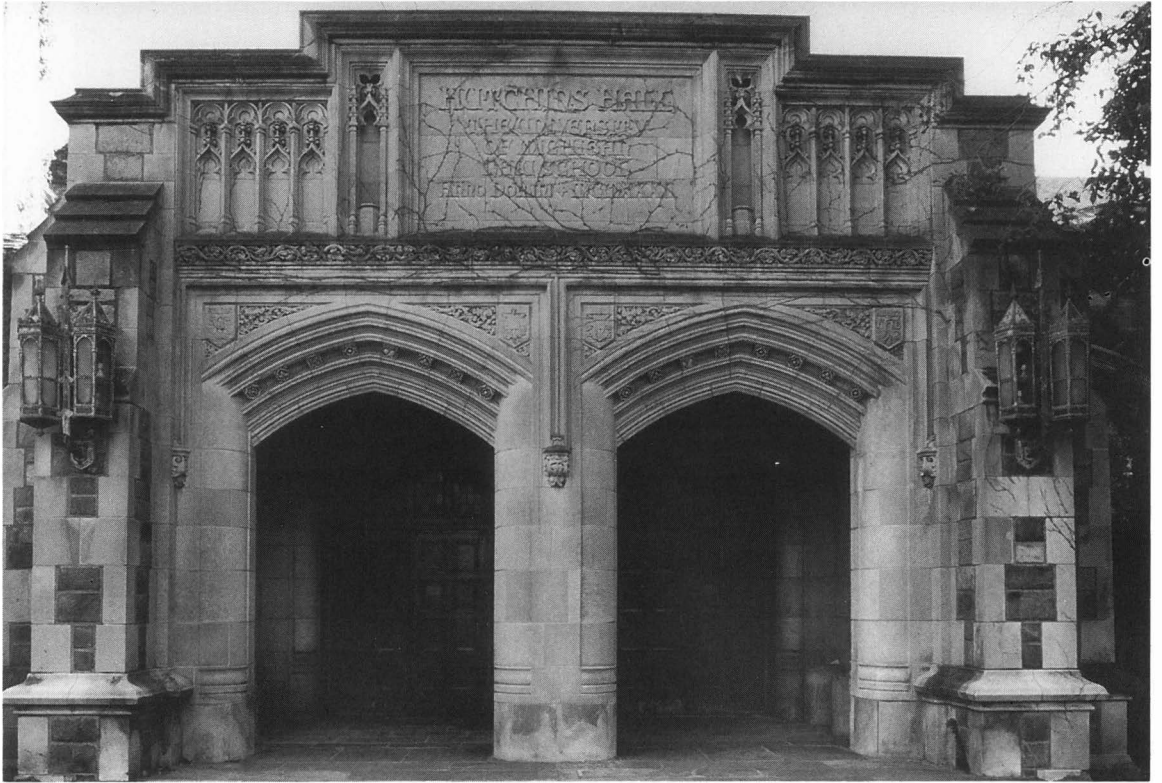
Fig. 35. Hutchins Hall, north entrance from the courtyard
