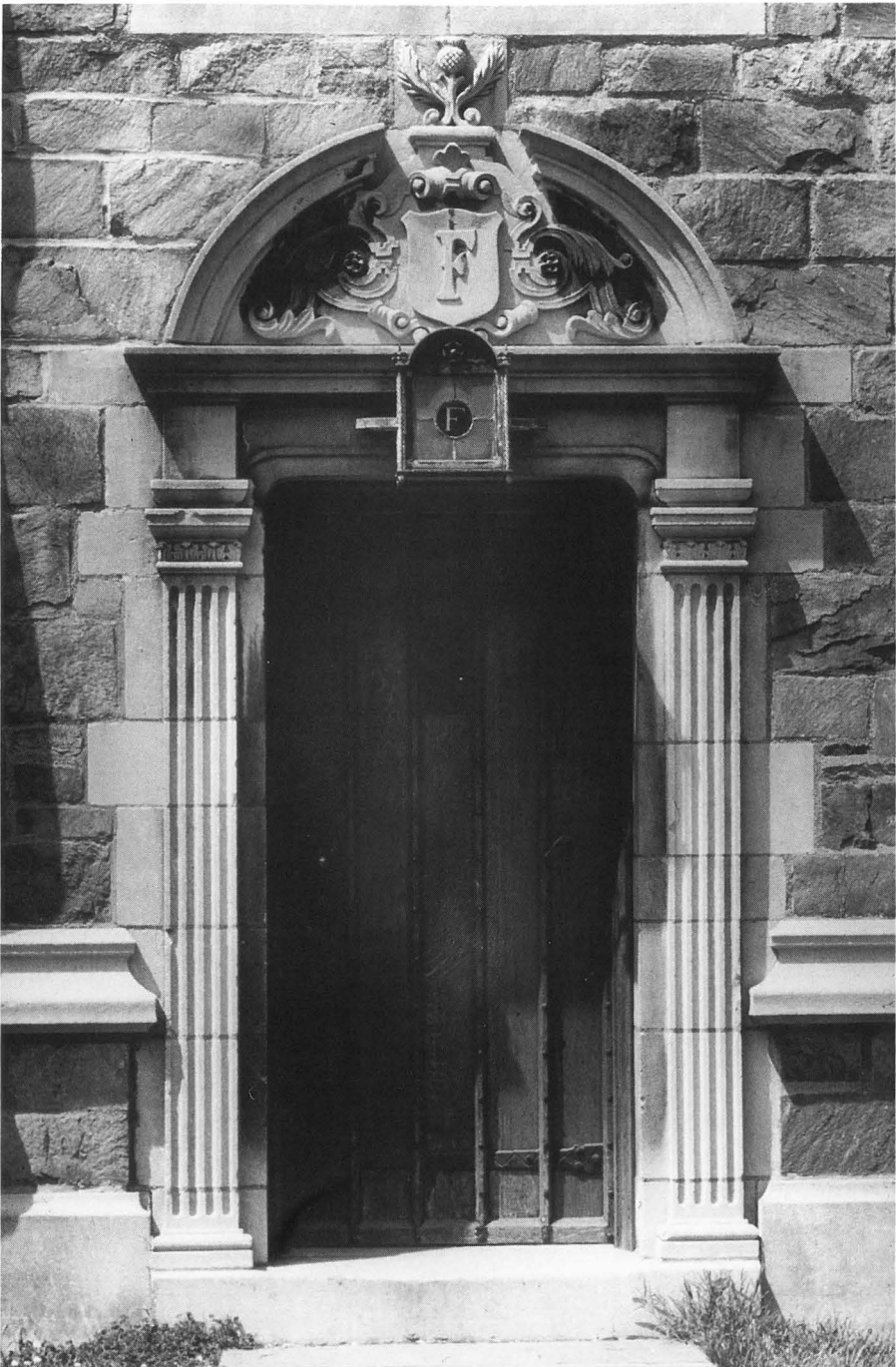
Fig. 26. Law Quad, stonework and entries on the courtyard
