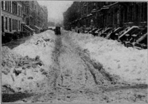
STREET NEARLY IMPASSABLE—SNOW PILED ON SIDES
