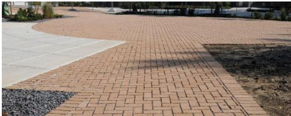
Figure 3: An example of a permeable pavement installation [6]
