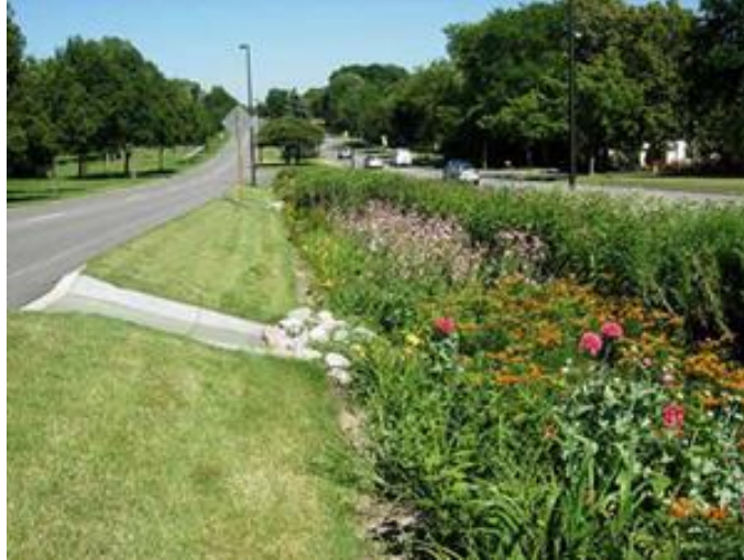
Figure 2: An example of a roadside bioswale [6].
