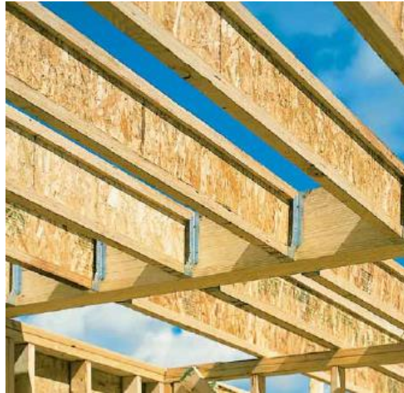
Figure 16: I-joists utilized in combination with glulam beams [9].
