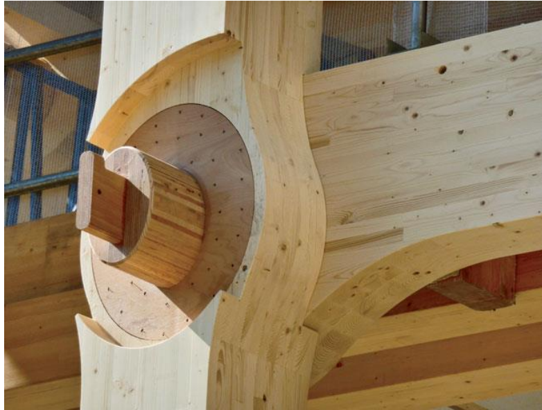
Figure 24: Joint detail with exposed plywood connection element [23].
