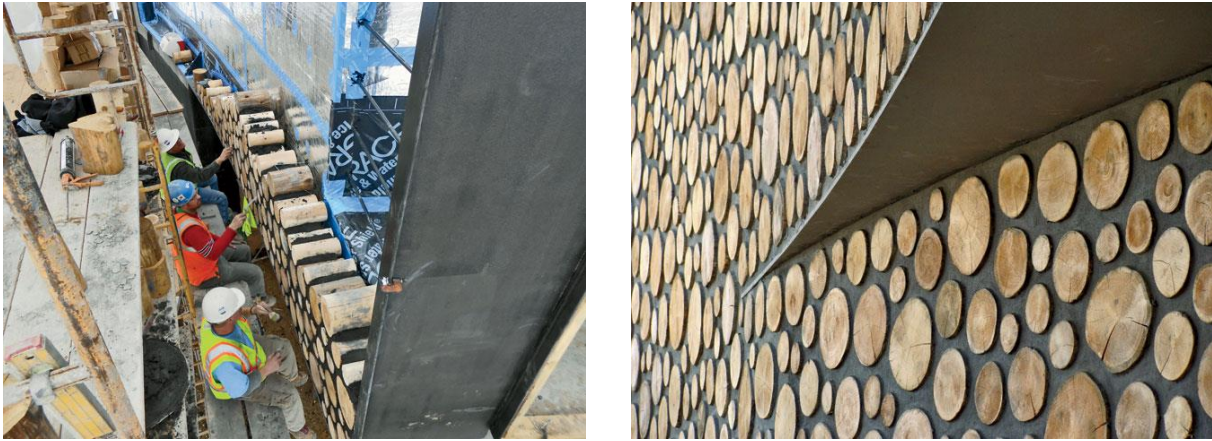
Figure 32: Logs of various diameter were carefully placed to provide even distribution [25].
