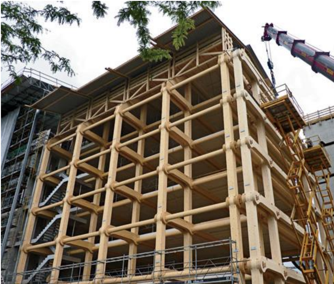
Figure 23: Timber structure prior to curtain wall installation [23].
