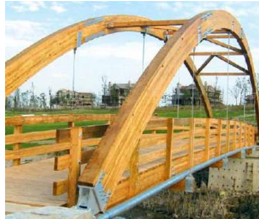
Figure 8: Bridge with custom glulam members [9].
