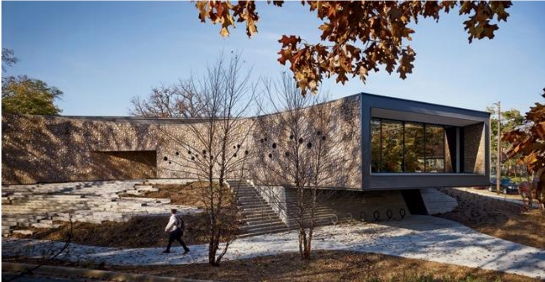
Figure 31: Cantilevered portion of the Arcus Center [27].
