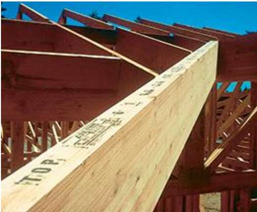
Figure 7: Truss with unbalanced glulam members [7].
