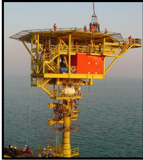
Figure 12 - Finished monopole offshore structure after installation. [Photo courtesy of Dr. Anil Patnaik, The University of Akron]
