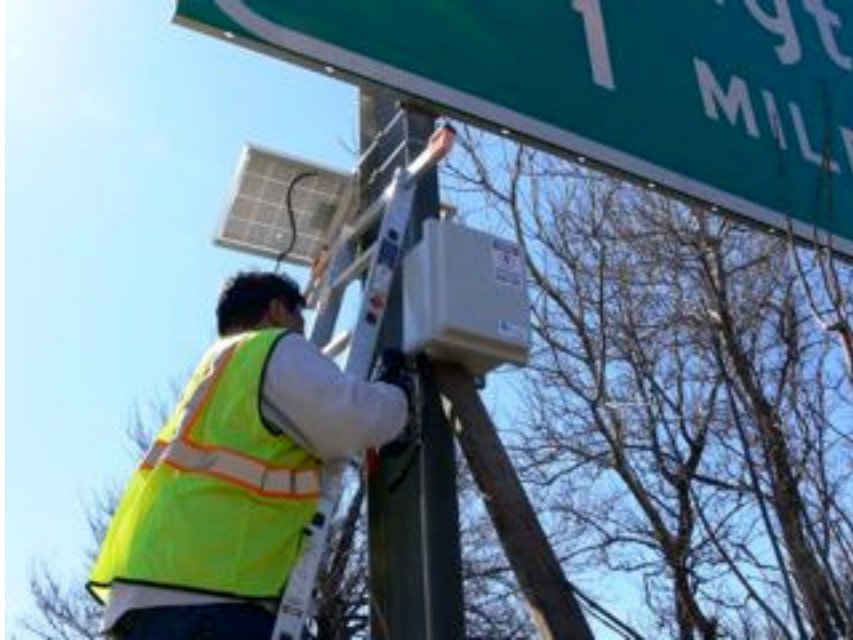
Figure 9: Trafficast's BlueTOAD Installation (Trafficast, 2012)
