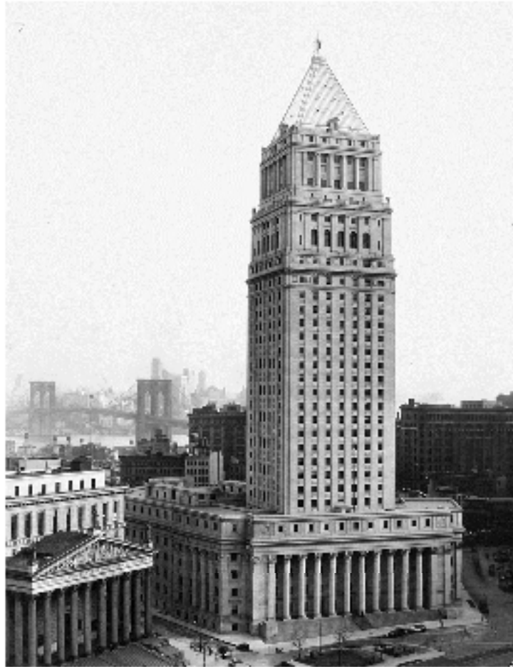
Figure 18: United States Courthouse, New York City, New York. Architect: Cass Gilbert, 1936; renamed in 2001 the Thurgood Marshall United States Courthouse.
