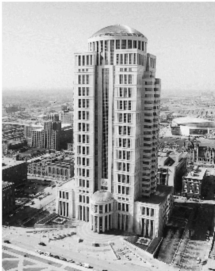
Figure 23: Thomas F. Eagleton Federal Courthouse, St. Louis, Missouri. Architects: Hellmuth, Obata + Kassabaum Inc., 2000.
