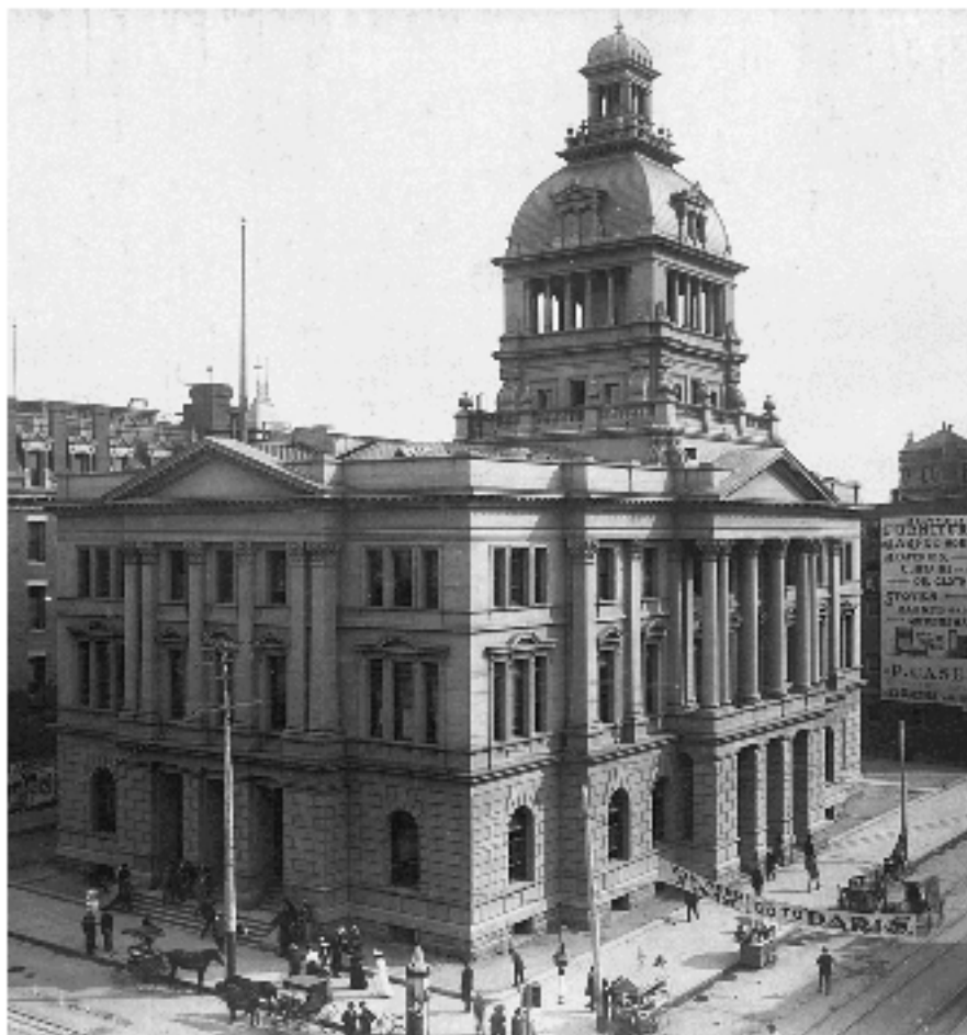
Figure 12: United States Post Office at 16th (Sixteenth) and Arapahoe Streets, Denver, Colorado. Supervising Architects: Mifflin E. Bell and Will. A. Freret. 1892.
