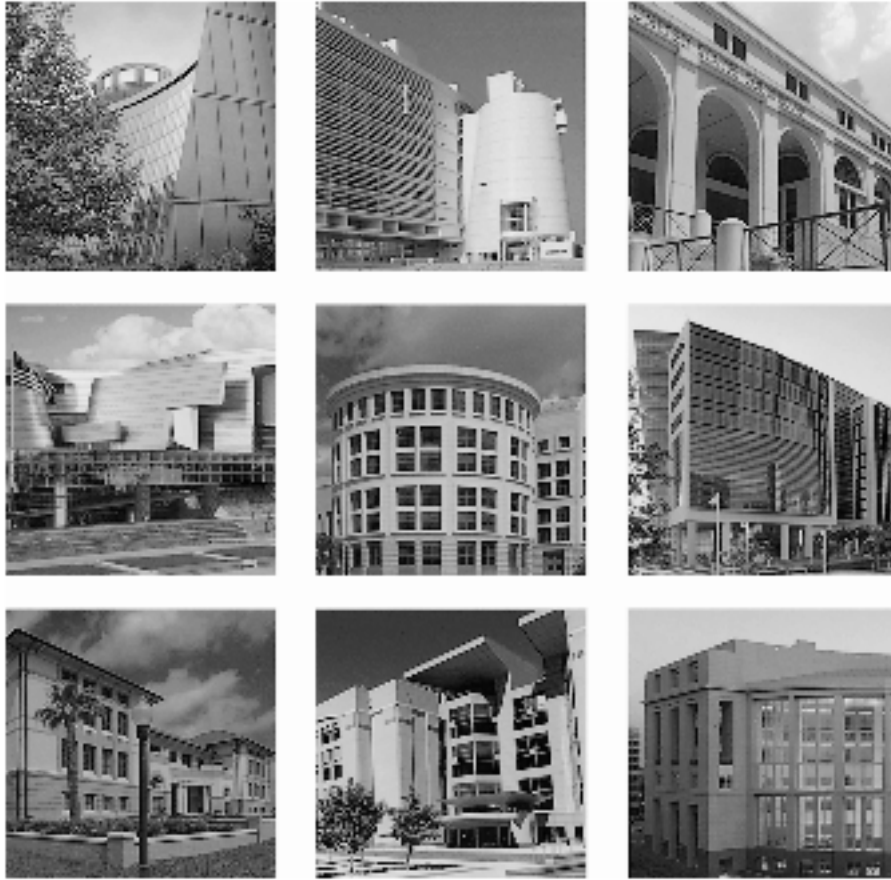
Figure 28: United States Courthouse Buildings and Renovations: A Sampling, 1998–2002. Photographs taken by Taylor Lednum, Thomas Grooms, and Frank Ooms, and provided courtesy of the Design Excellence Program, Office of the Chief Architect, United States General Services Administration. From the top, moving left to right, the courthouses and their architects are John Joseph Moakley U.S. Courthouse (Boston, Massachusetts), designed by Henry Cobb of Pei Cobb Freed & Partners Architects LLP and Jung/Brannen Associates, completed 1998; Alfonse D’Amato U.S. Courthouse (Central Islip, New York), designed by Richard Meier & Partners and The Spector Group, completed 2000; United States Courthouse (Tallahassee, Florida), designed by Reynolds Smith and Hills Inc. and William Morgan Architects, completed 1999; Wayne Lyman Morse United States Courthouse (Eugene, Oregon), designed by Morphosis and DLR Group, completed 2006; William B. Bryant United States Courthouse Annex (Washington, D.C.), designed by Michael Graves & Associates and SmithGroup, completed 2005; Wilkie D. Ferguson United States Federal Courthouse (Miami, Florida), designed by Arquitectonica and Hellmuth, Obata + Kassabaum Inc., completed 2007; Corpus Christi Federal Courthouse (Corpus Christi, Texas), designed by Hartman-Cox Architects, William S. McCord—AIA-Principal/Architect of Record, and WKMC Architects Inc., completed 2001; the Roman L. Hruska U.S. Courthouse (Omaha, Nebraska), designed by Pei Cobb Freed & Partners and DLR Group, completed 2000; and Spottswood W. Robinson III and Robert R. Merhige Jr. Federal Courthouse (Richmond, Virginia), designed by Robert A.M. Stern Architects and HLM Design, completed 2008.
