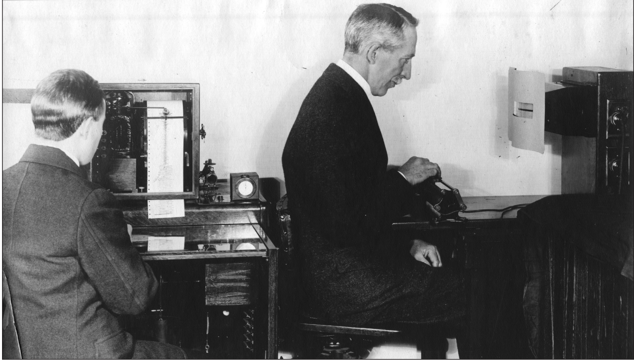
Figure 2. The pursuit meter, created by Miles to measure hand-eye coordination.
