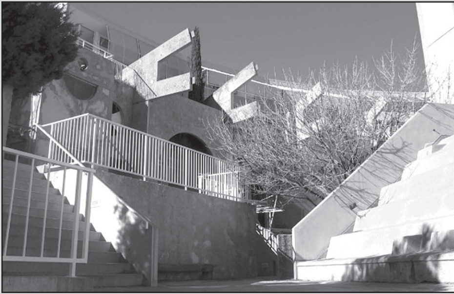
THE EAST CRESCENT (FACADE) OF ARCOSANTI
