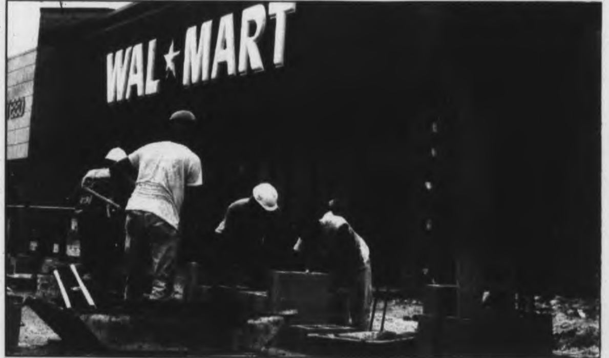
Workers from McIntosh Masonery, Richmond, laid blocks on the new Super Wal-Mart. Construction is expected to be completed sometime before Christmas.
