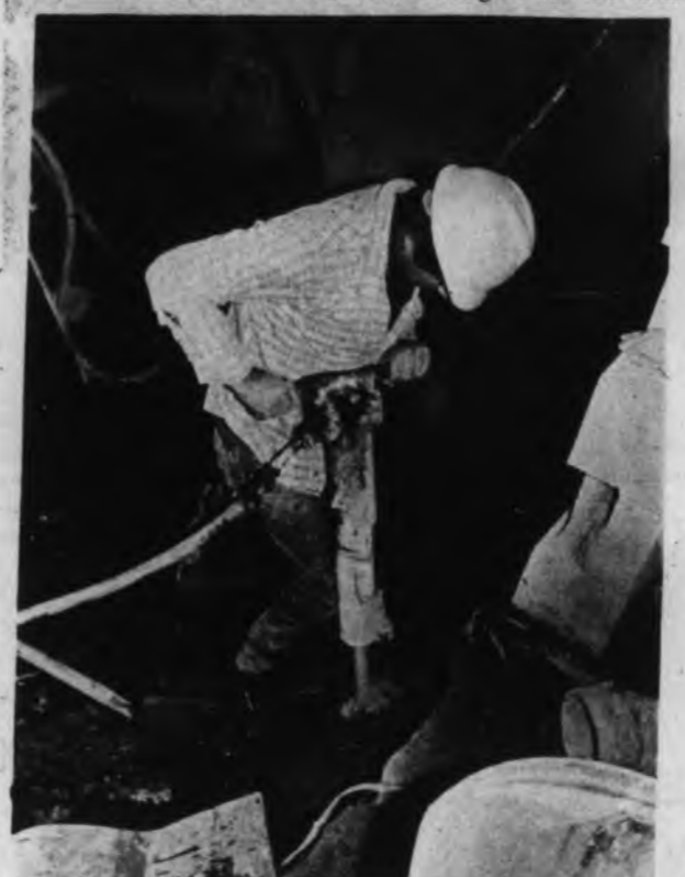
Getting down to a somewhat muddy job a workman breaks up concrete so that an elevator can eventually be installed while a fellow worker removes some old venetian blinds
