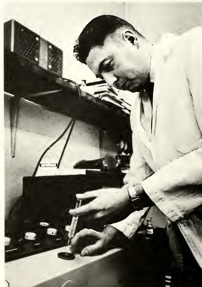
Dr. John Meisenheimer introduces a liquid sample into a gas chromatograph to obtain information that will be of great help in his research project on the synthesis of biologically active organic compounds.
