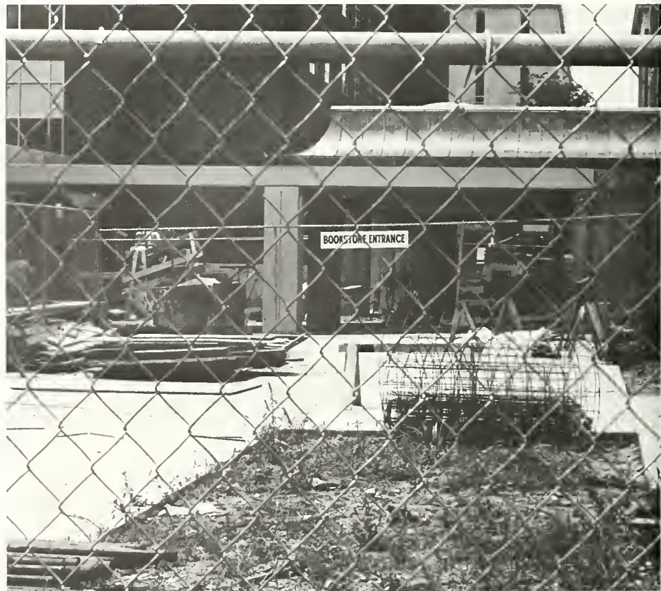
Fences enclose the University store and Jane F. Campbell Building during construction.
