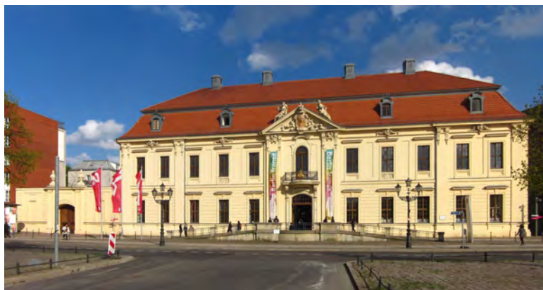
View of Collegienhaus from Lindenstrasse.
