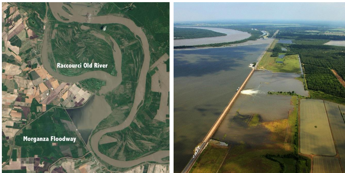
Fig. 6. NASA and USACE photos of the Floodway in May 2011 (Wikipedia Commons, USACE).
