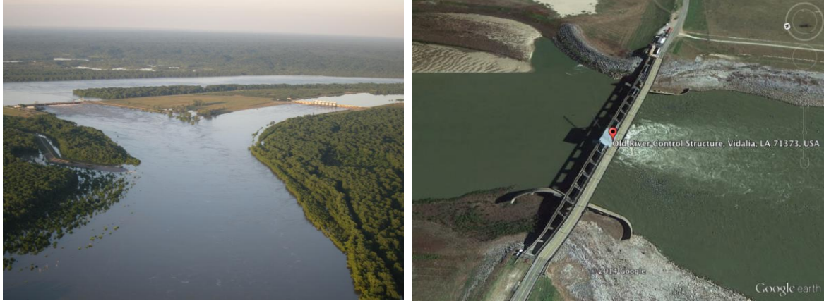
Fig. 7. Lower Auxiliary Structure at Old River (personal photo), ORCS via USACE Flickr and GoogleEarth.
