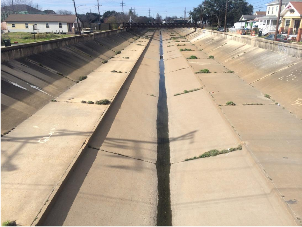
13. Near-empty drainage canal in Broadmoor neighborhood, New Orleans.
