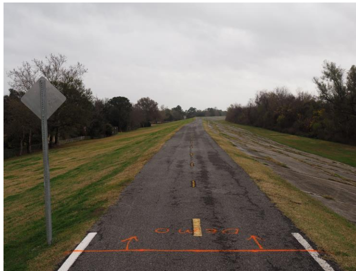
Fig. 3. The levee at Sauv e's Crevasse (personal photo).
