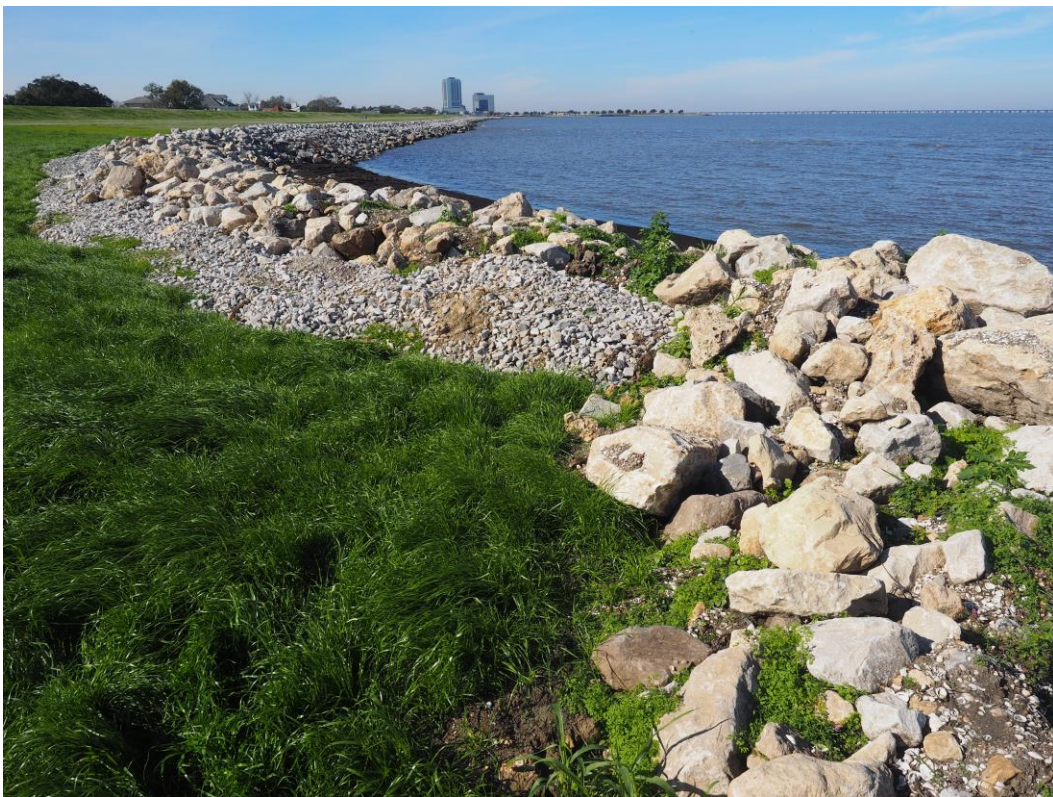
10. Stone levee at Bucktown Harbor on Lake Pontchartrain, New Orleans.
