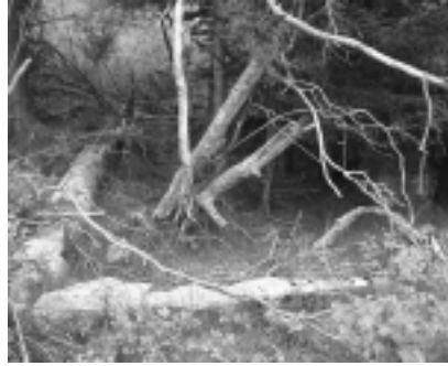
Overgrown foundation of side of main house.
