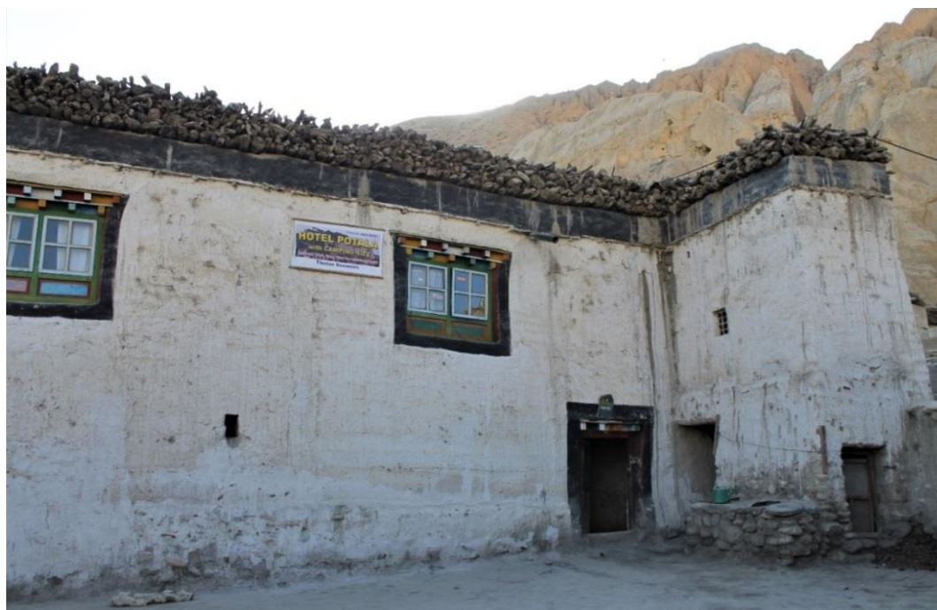
Figure 3.22. A lodge locally constructed from stone and baked mud bricks in Surkhang (Date: June 2018, Source: Author)
