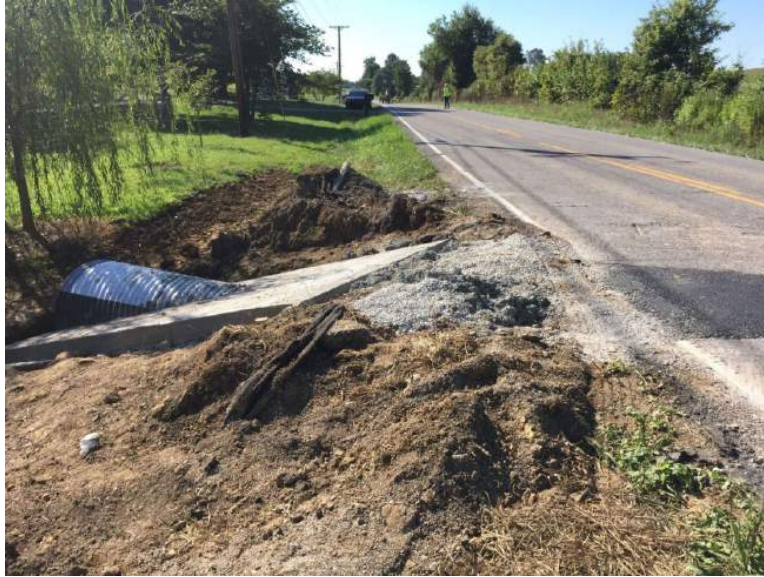
Figure 1 Headwall Installed on a Skew at STA 170+76 RT
