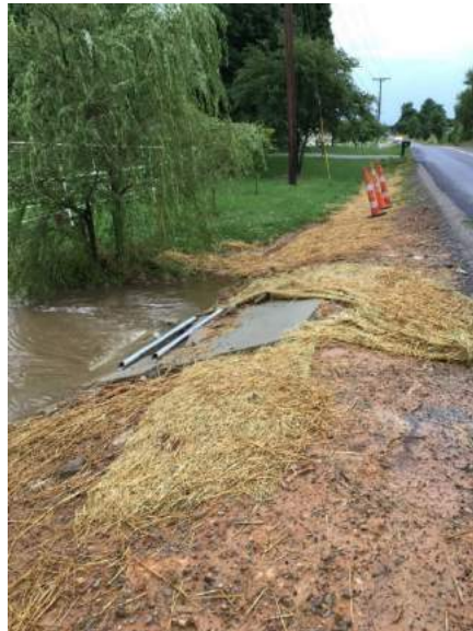
Figure 2 Reconstructed Headwall at STA 170+76 RT
