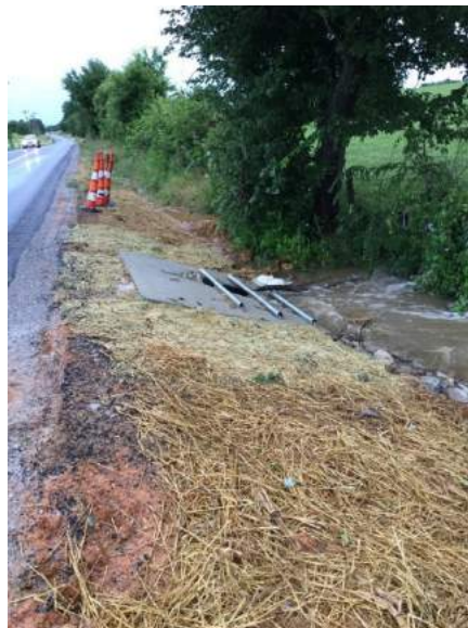
Figure 5 Grate Bars on 36-inch Sloped and Mitered Concrete Headwall
