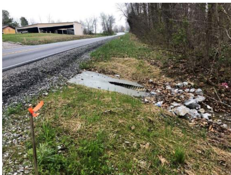
Figure 7 New Headwall and Improvements to the Clear Zone
