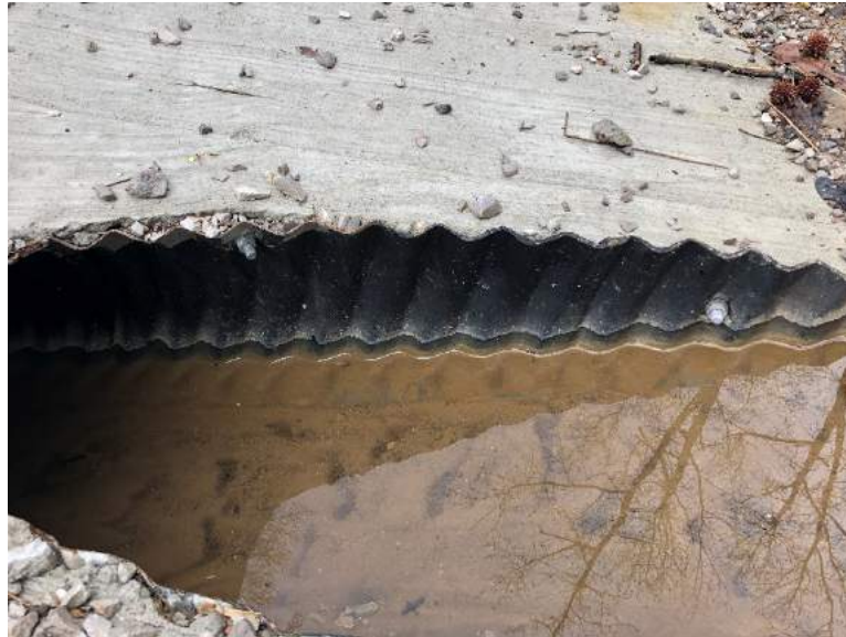
Figure 8 Mitered Pipe End Secured to Headwall
