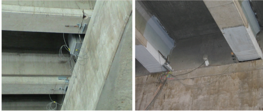
Figure 6. Instrumentation on Beams 6 and 7 before and after strengthening with CFRP sheets/fabric.
