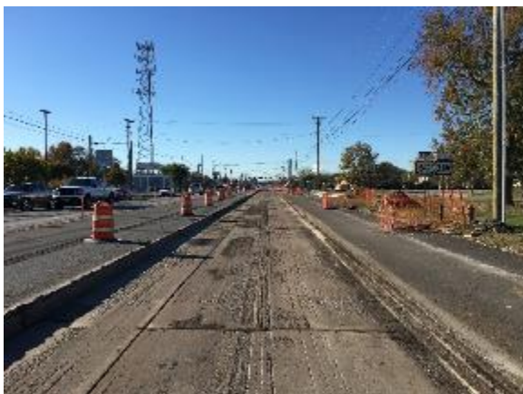
Figure 17 Pavement Prepped for Fabric
