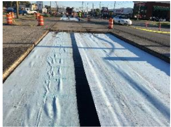
Figure 13 Piecemeal Installation
