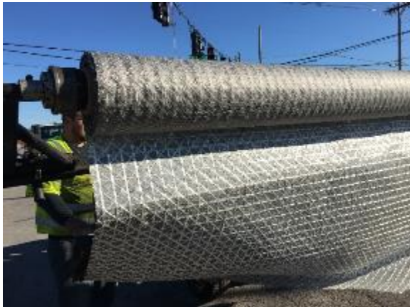
Figure 21 Close-Up of Paving Grid
