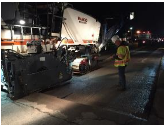
Figure 6 Pavement Milling Process
