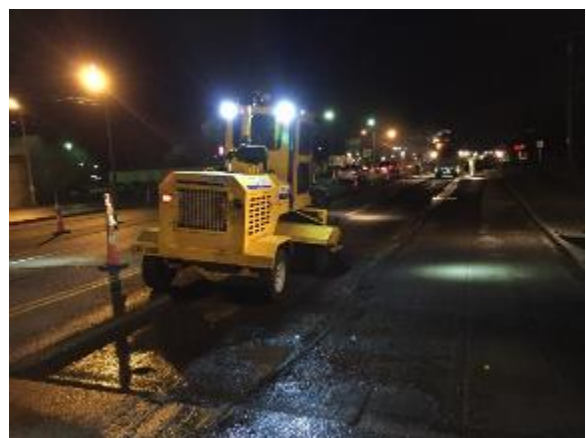
Figure 5 Pavement Prep For RCRI
