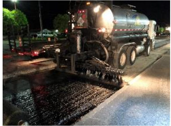
Figure 24 Applying Tack Coat as Adhesive
