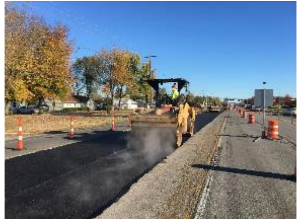
Figure 22 Compaction of Base Course
