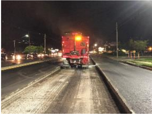
Figure 23 Pavement Prep for Paving Grid
