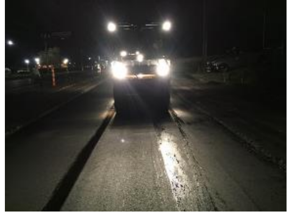
Figure 8 Compaction of RCRI
