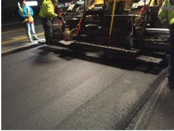
Figure 7 Placement of RCRI
