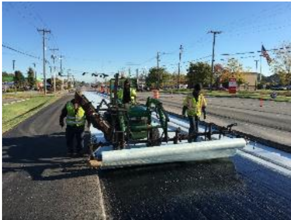
Figure 12 Fabric Placement
