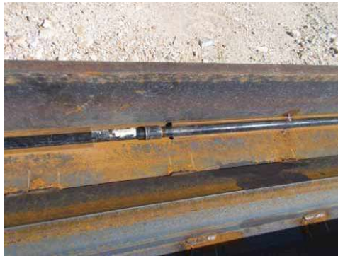
Figure 35. H-Pile Load Tell Tale Housing
