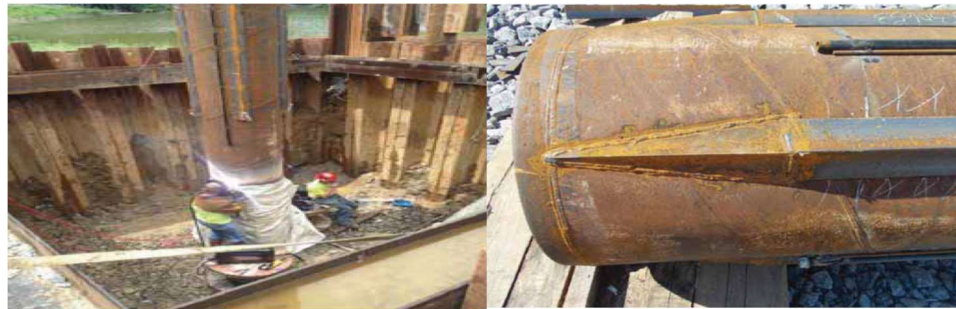
Figure 14. Pipe Pile Instrumentation: (a) Pile Splicing; (b) Driving Shoe
