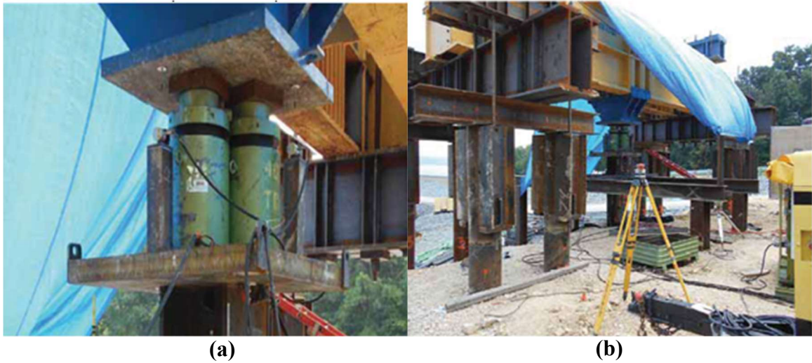
Figure 16. Static Load Test Equipment: (a) Hydraulic Jacks; (b) Load Test Frame
