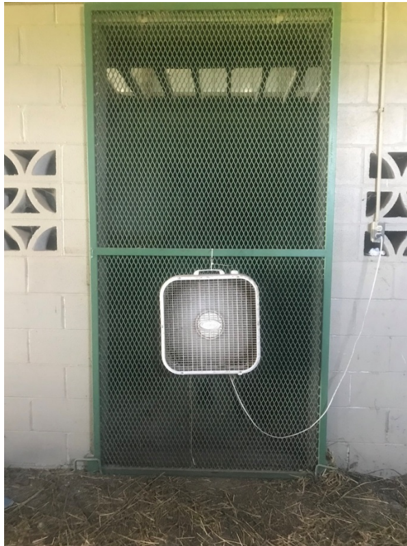
Figure 2.7 Position of fan for lower fan placements.
