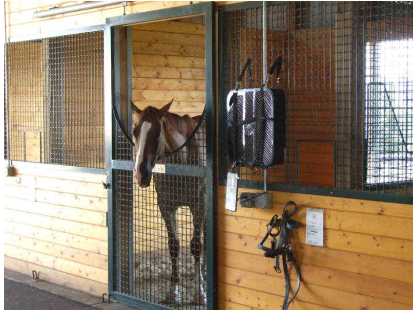
Figure 2.3 Stall wall fan that blew into and out of the stall.
