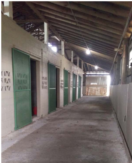
Figure 2.5 Layout of barn for Year 2. Aisle way along the outside of the barn with the stalls in the center of the barn and concrete block walls. The aisle way door (closed in this image) that can be opened to allow air to move down the aisle is at the far end of the image.
