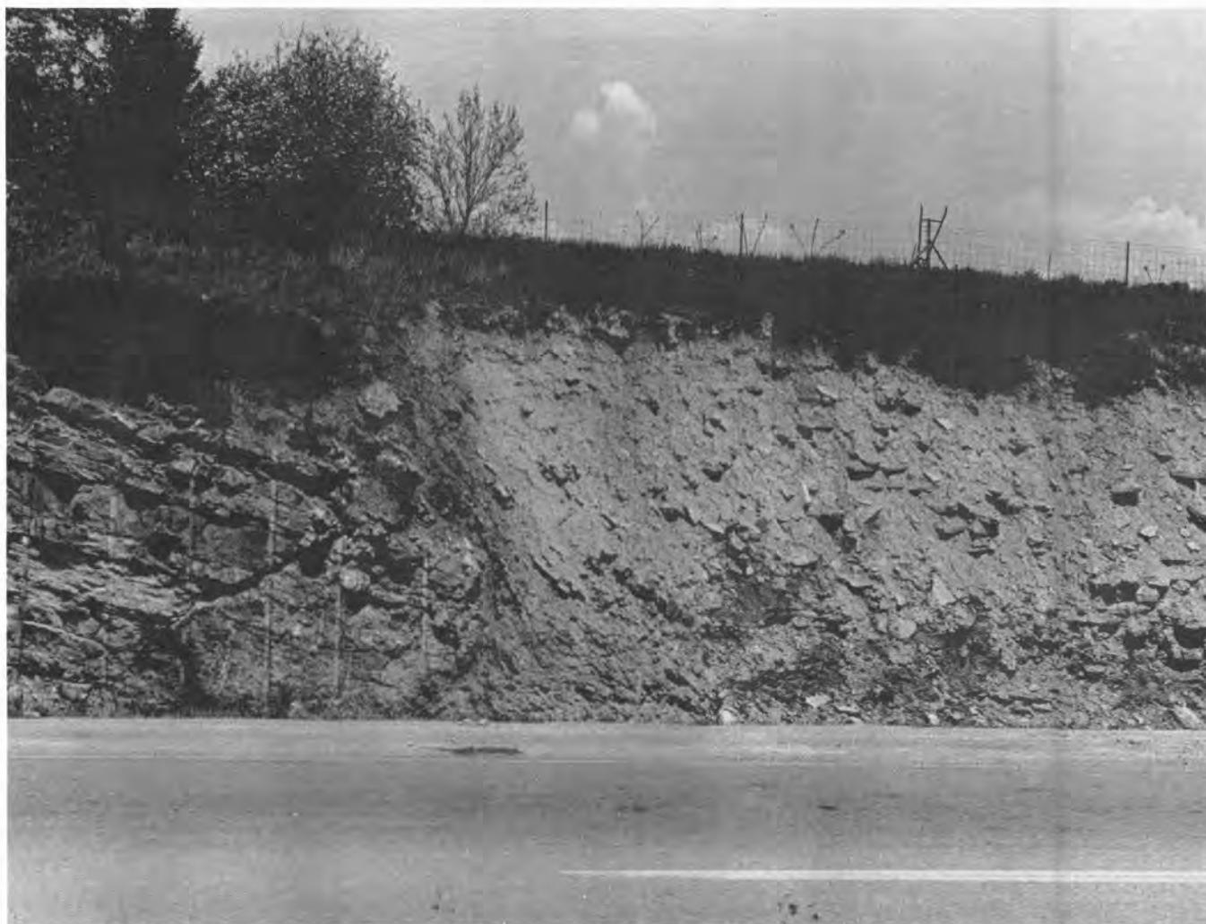
Figure 2. Lexington Fault System along U. S. Highway 68 Bypass, north of Paris, Bourbon County. The Marsh Vein is exposed in the limestones on the left side of the fault.
