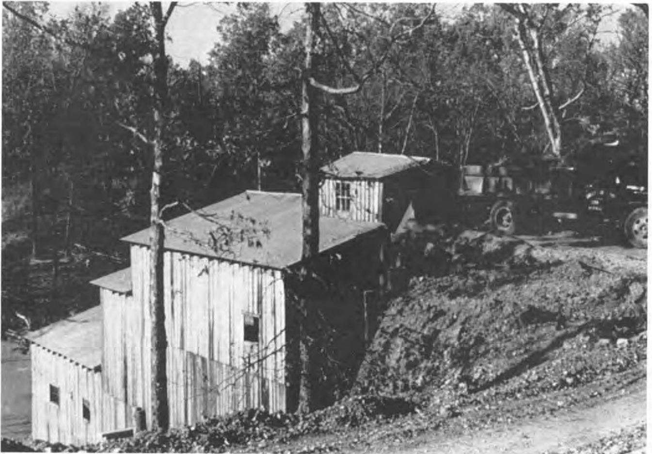
Figure 19. Barite concentration mill at Mico Mine in 1958.
