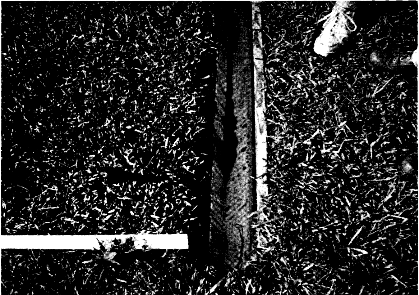
Figure 5. Gutter below filter strip.
