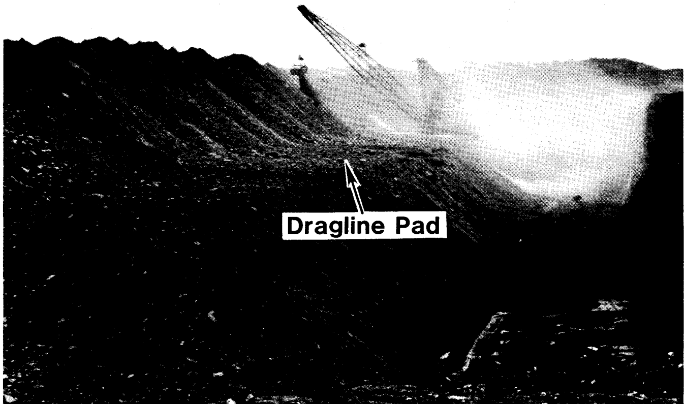
Figure 7. Dragline pad built on spoil.
