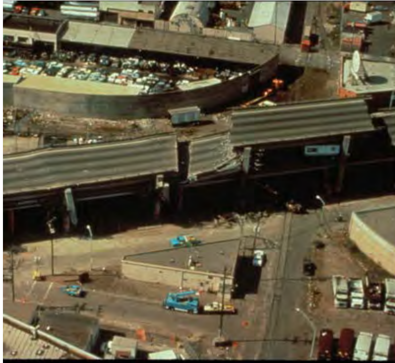
Figure 1-4. I-80 damage during the 1989 Loma Prieta earthquake.
