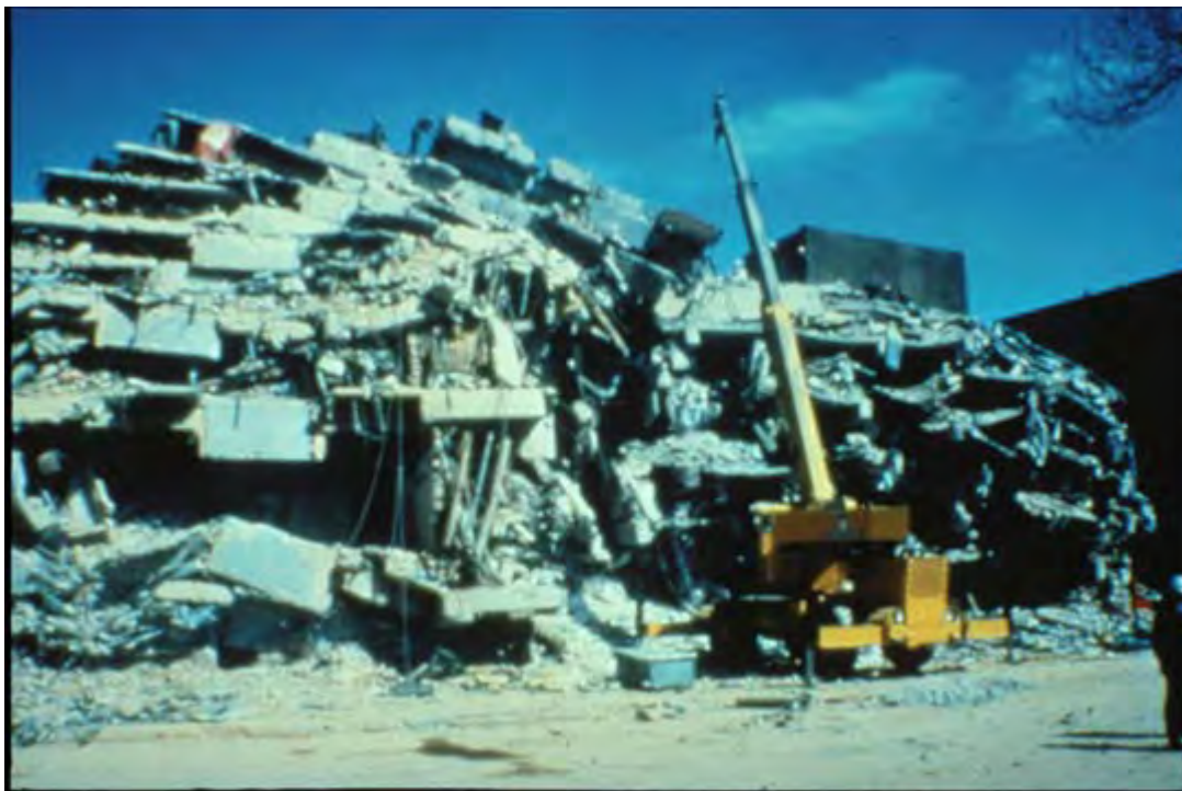
Figure 1-5. Complete destruction of a building caused by amplified ground motion in Mexico City during the 1985 Mexico earthquake.
