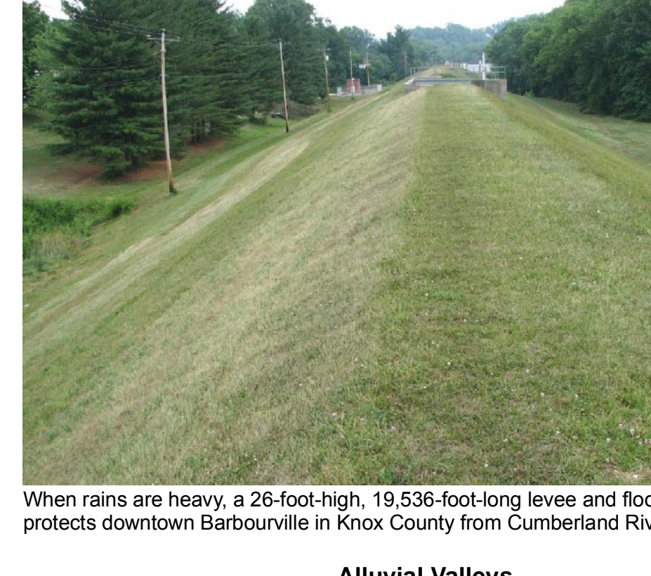
When rains are heavy, a 26-foot-high, 19,536-foot-long levee and floodgate system protects downtown Barbourville in Knox County from Cumberland River flooding.
