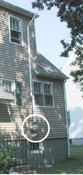
Ventilation system removes radon from the basement area of this home on unit 5. Photo by Dan Carey, Kentucky Geological Survey.
