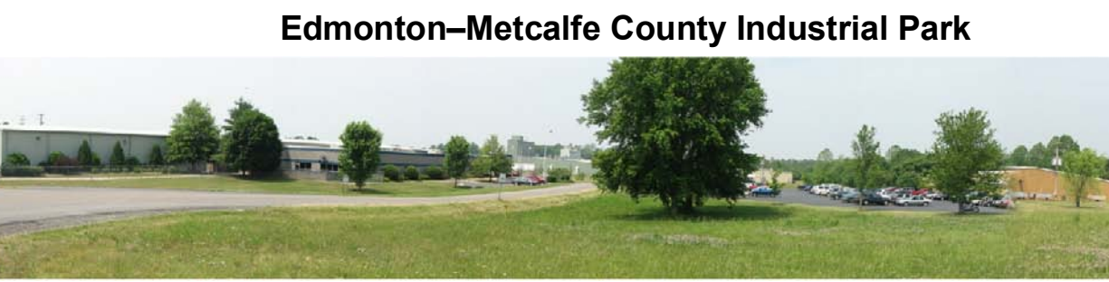
Transportation to and from the 7-acre Edmonton-Metcalfe County Industrial Park is provided by the Louise B. Nunn Parkway (below). Photos by Dan Carey, Kentucky Geological Survey.
